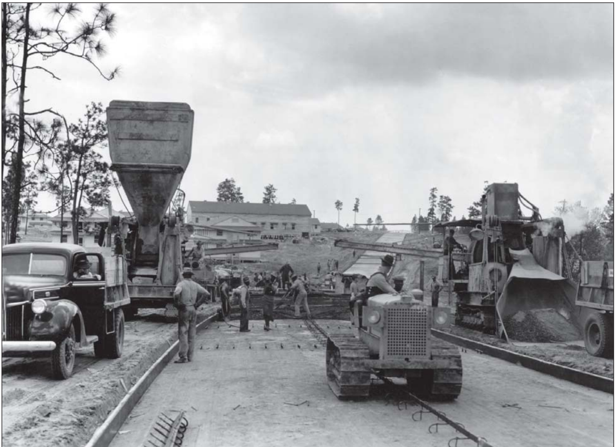
Camp Polk’s main road, Mississippi Avenue, under construction on April 30, 1941.
