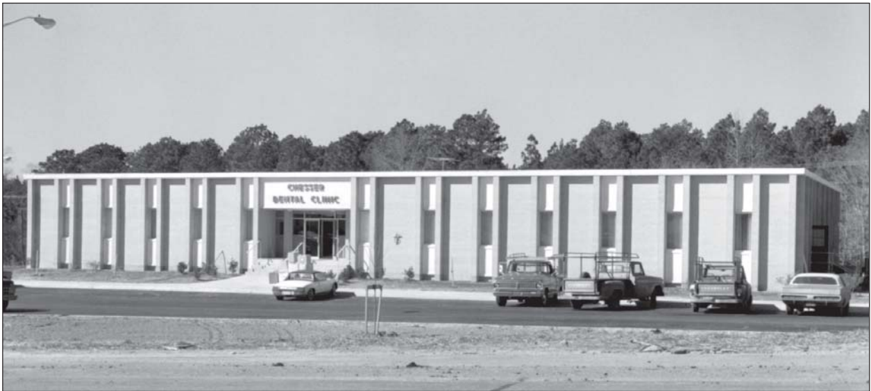
In an ongoing effort to ensure quality health care, the Army built the Chester Dental Clinic at Fort Polk in 1976.
