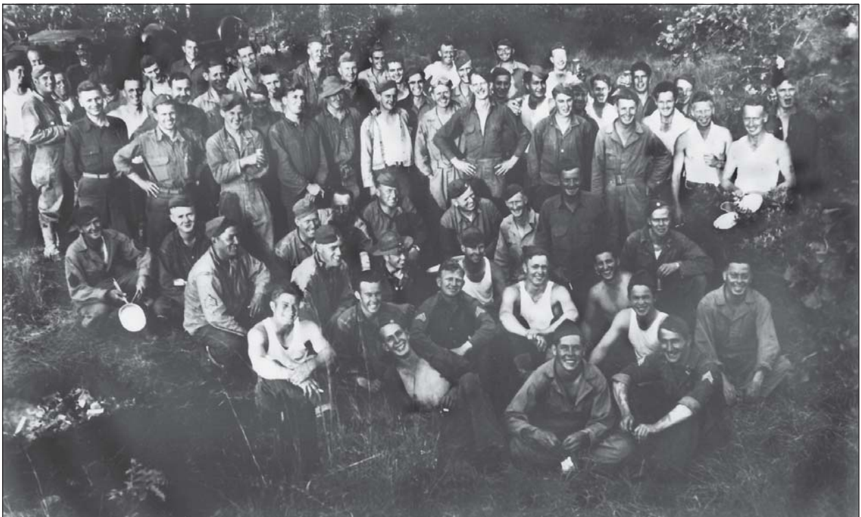
The Louisiana Maneuvers tested all aspects of the U.S. military, including how soldiers would handle building roads, bridges, and camps for thousands of troops. An 11th Infantry convoy (top) crosses one of the pontoon bridges built during the maneuvers, and men from the 7th Engineers, Company A (bottom), take a break from construction labors.
